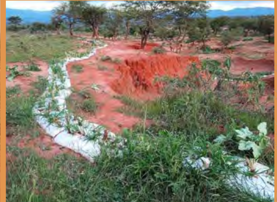
Vetiver splits planted in soil bags along the contour lines
