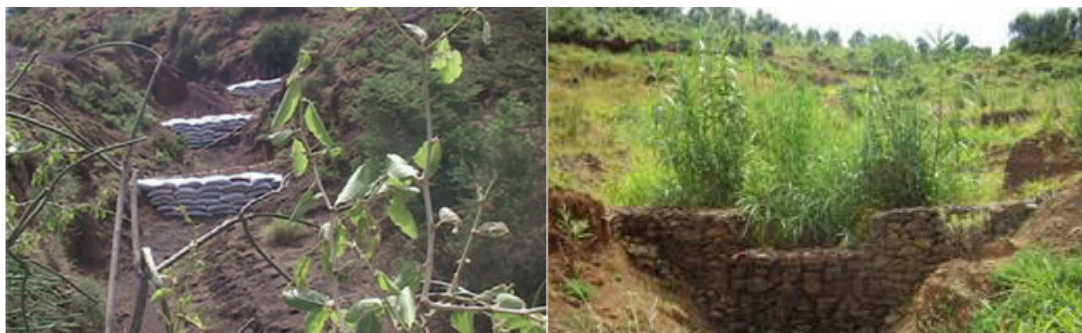
Plate 16. Sandbags (left) and a gabion (right) constructed across a gully.
