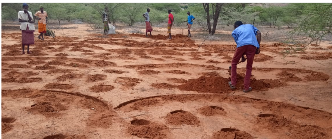
Plate 12. Creating micro-water catchment structure under FMNR practice by communities in Marsabit, Kenya Photo: CARE Somalia
