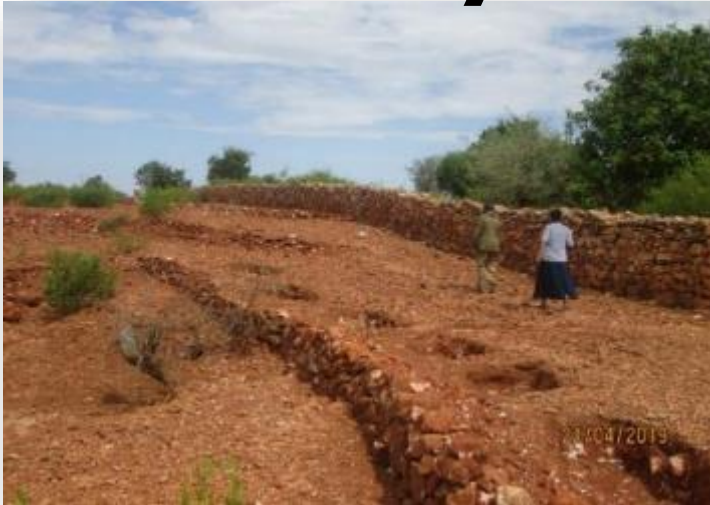
Moisture retention structure for greening in dry and degraded areas of Asgedetsimbela site, Woreda/ region. Photo: Asfaw Mariame
