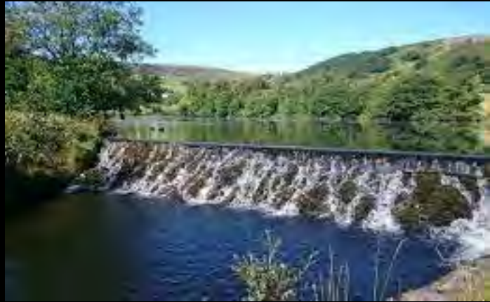
Conservation of major water towers in Kenya.
