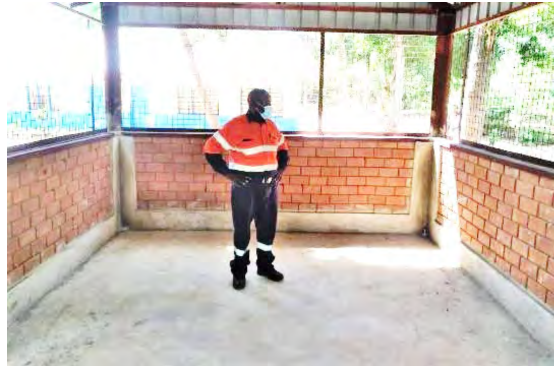
Renovation of a school kitchen using Base interlocking blocks
